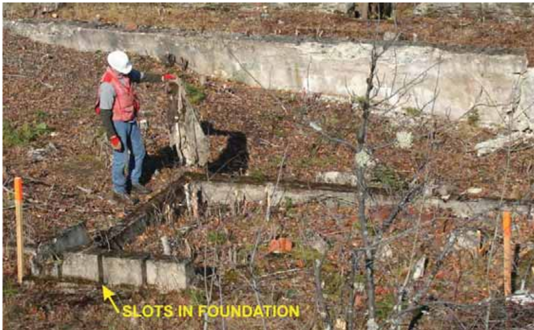
Figure 2.26. Slots in part of the foundation of the Stone Wall residence.
