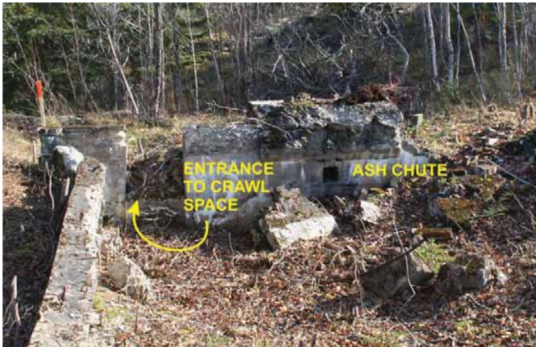
Figure 2.25. Photograph of Stone Wall residence ash chute and entrance to crawl space.
