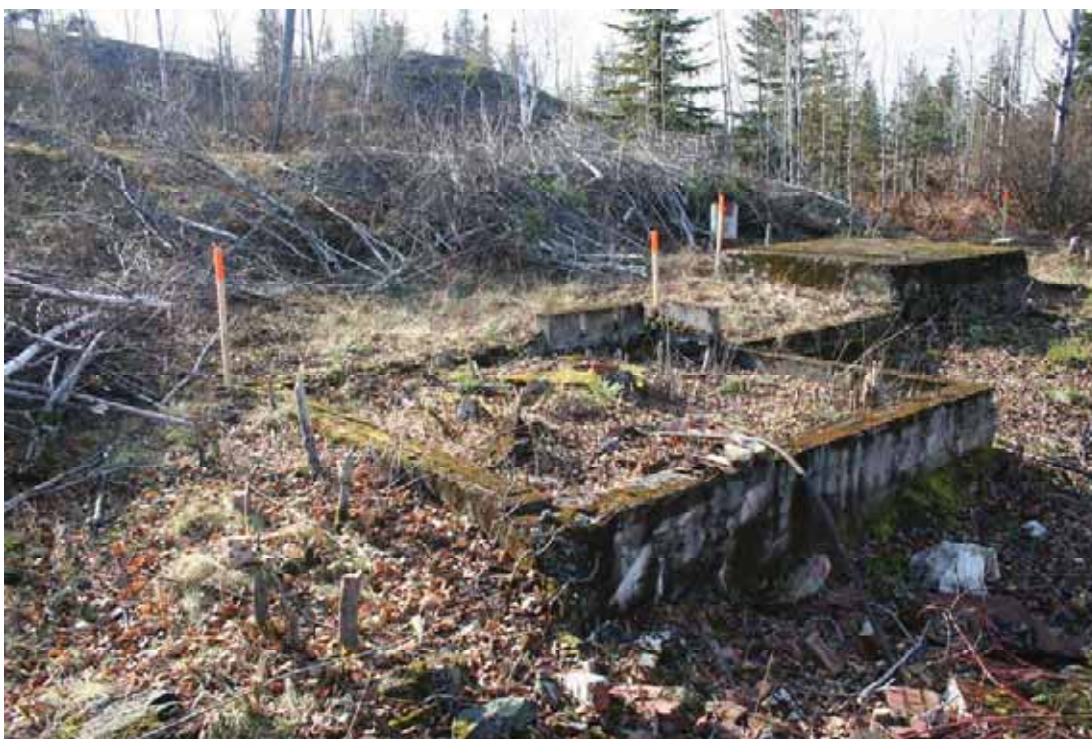
Figure 2.17. Photograph of kitchen/bath foundation.
