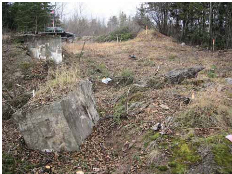
Figure 2.13. Photograph of two piers of the Manager's House foundation.
