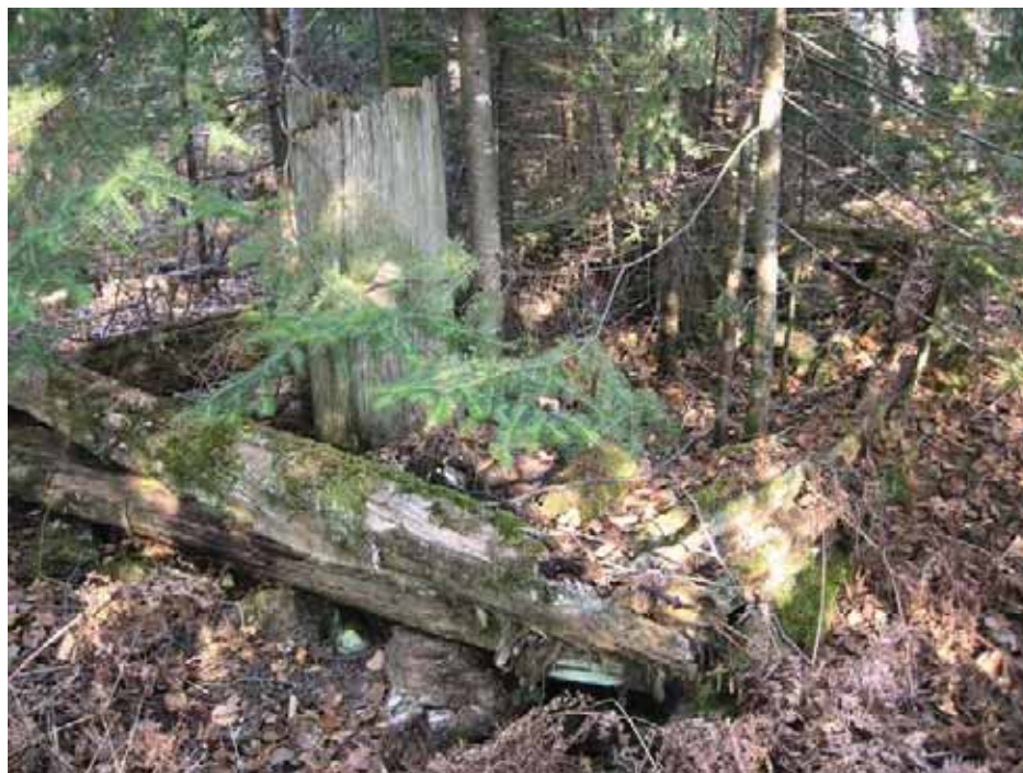
Figure 2.35. Photograph within the CPZ1 area showing an anchor pole support with cribbing.
