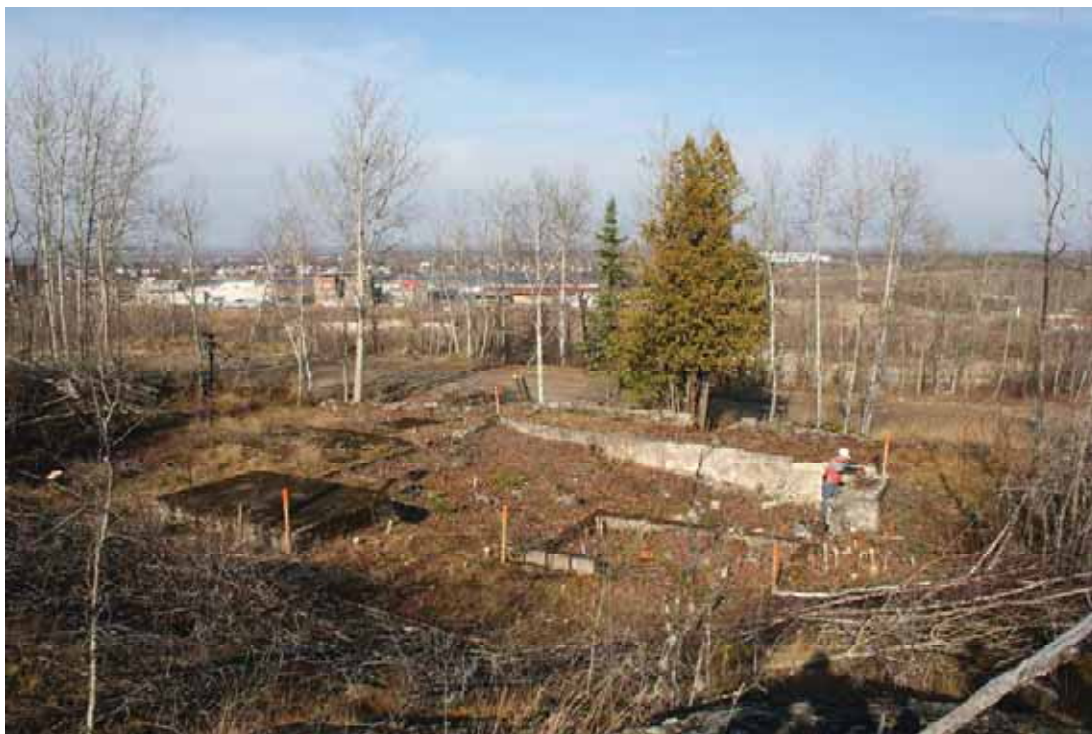
Figure 2.16. Photograph of the foundation of the Stone Wall residence.
