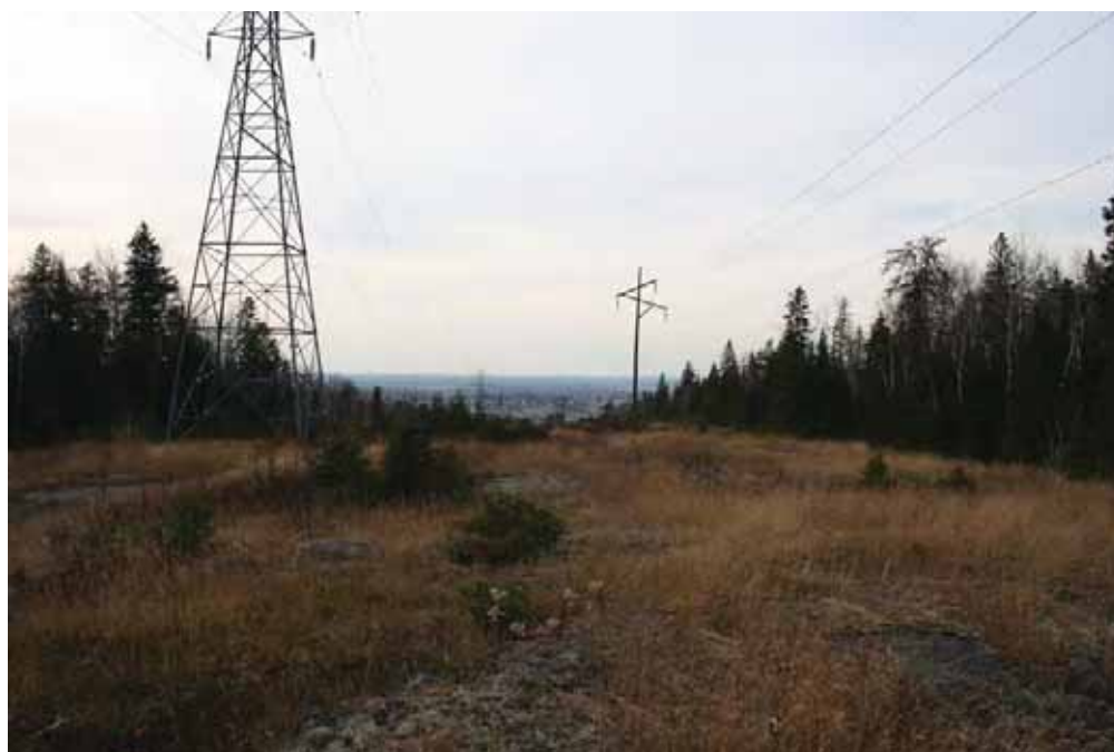
Figure 2.53. Photograph looking north along the east-west haul road corridor.
