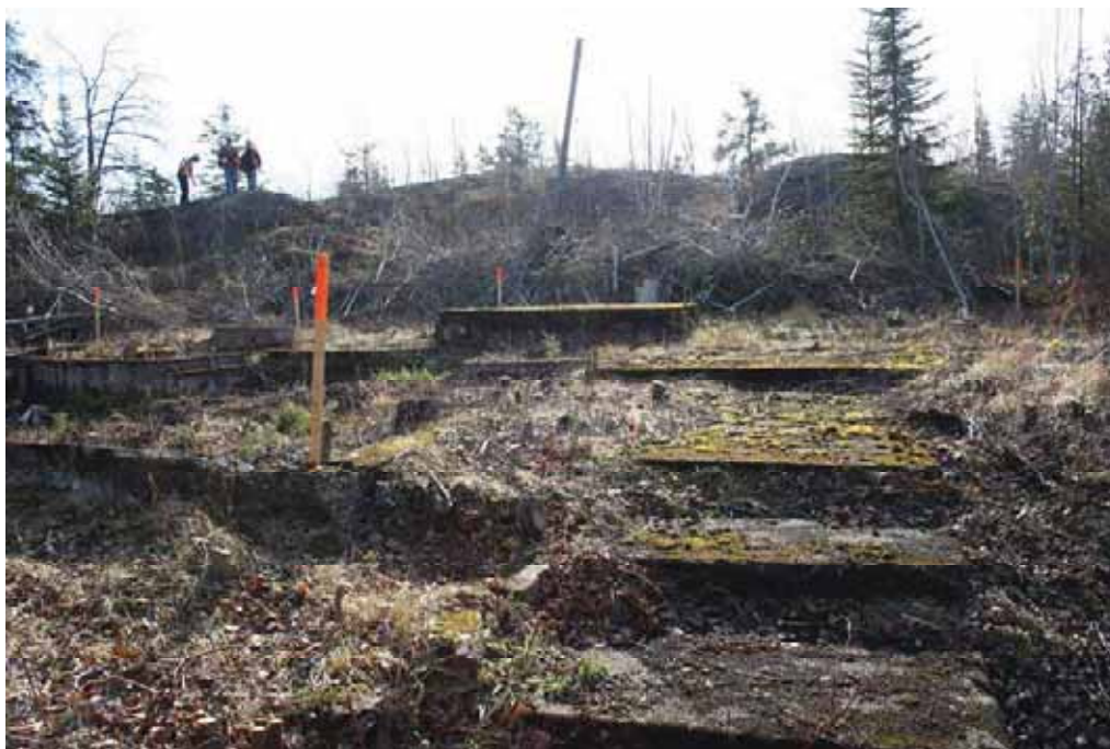
Figure 2.19. Photograph looking south at the poured concrete steps on the west side of the house. These steps lead up to a concrete patio area on the central right portion of the photograph.
