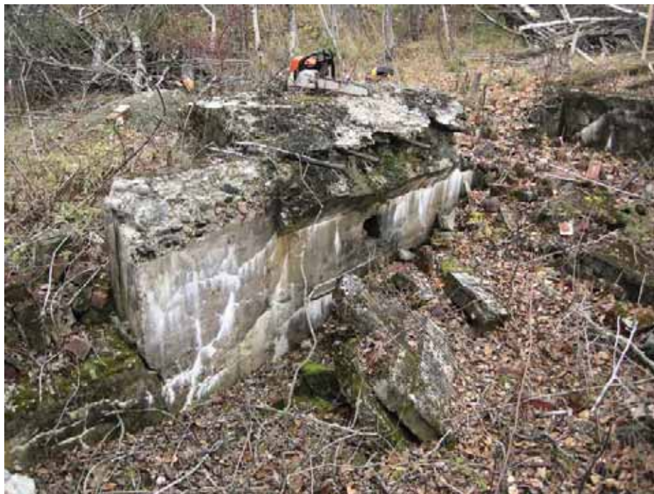
Figure 2.24. Remains of the fire place. Notice the drill steels and the ash chute.
