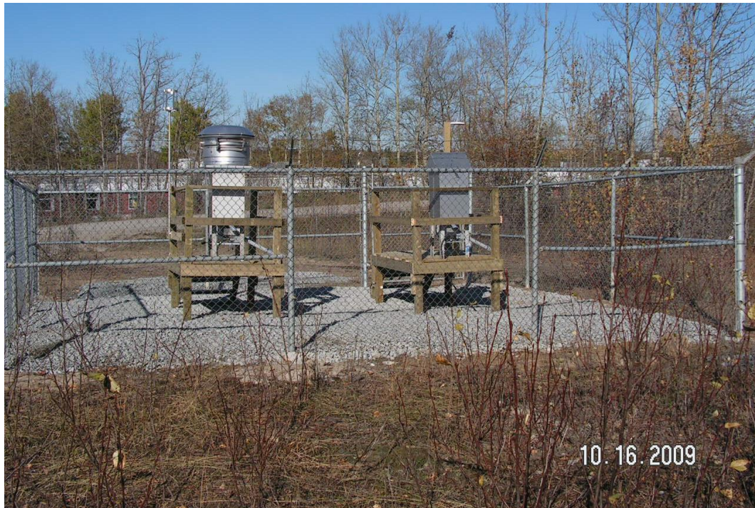
Figure 3: Photo of Air Sampling Station at the Extendicare Facility Site
